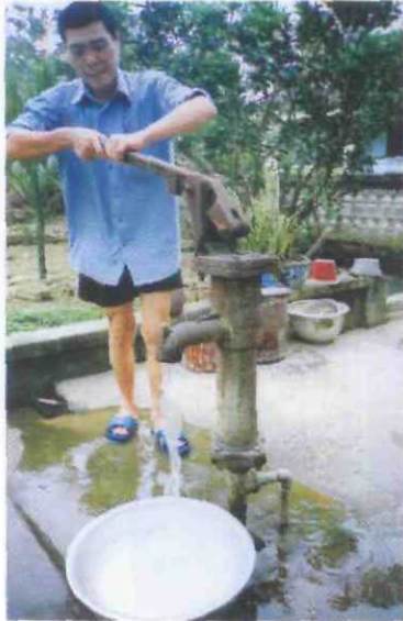
"No 6" water hand pump, adapted from those used in Bangladesh
